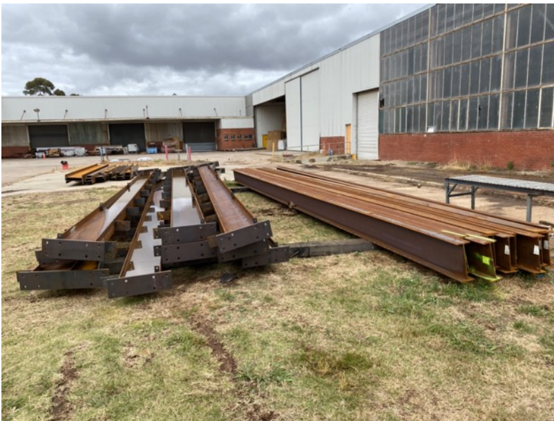
Photos (above): Local design and fabrication of the structural supports, ready for installation.
