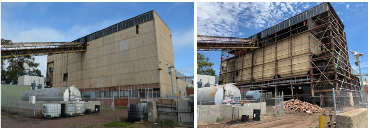
Photos (above): Before (left) and after (right) the asbestos cladding removal.
