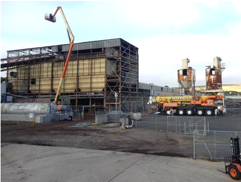
Photos (above): Legacy silos adjacent to the main building (left) being removed (right). One of the silos will be refurbished and repurposed for char storage & packing.
