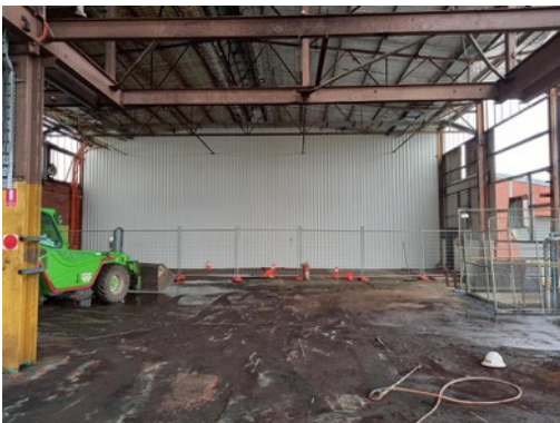
Photo (above): installation of a permanent partition wall to replace the temporary fencing that previously separated the plant area from the neighbouring tenant
