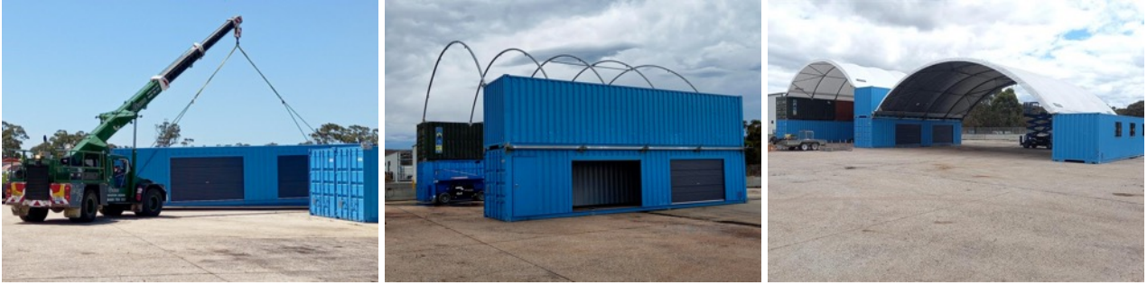
Photos (above): installation of the All Shelter structures designed to house the raw lignite, workshop and laboratory.
