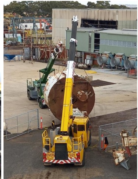
Photos (above): Legacy silos adjacent to the main building (left) being removed (right). One of the silos will be refurbished and repurposed for char storage & packing.
