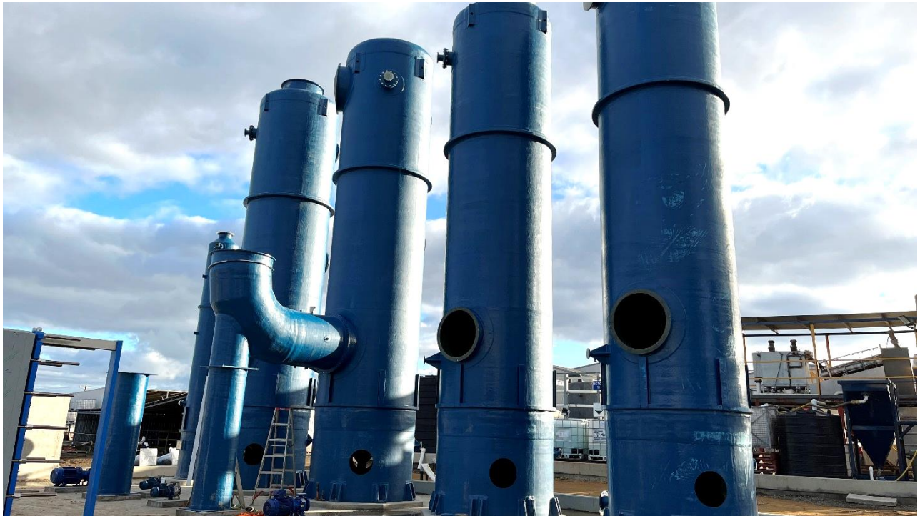
Installation of EVAPX® columns at the customer's site in New South Wales
