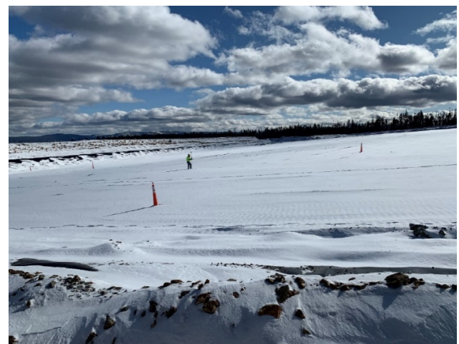
Dry stack tailings storage facility
