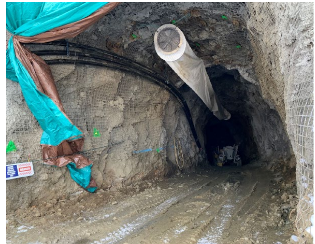
West Portal development with installed ventilation
