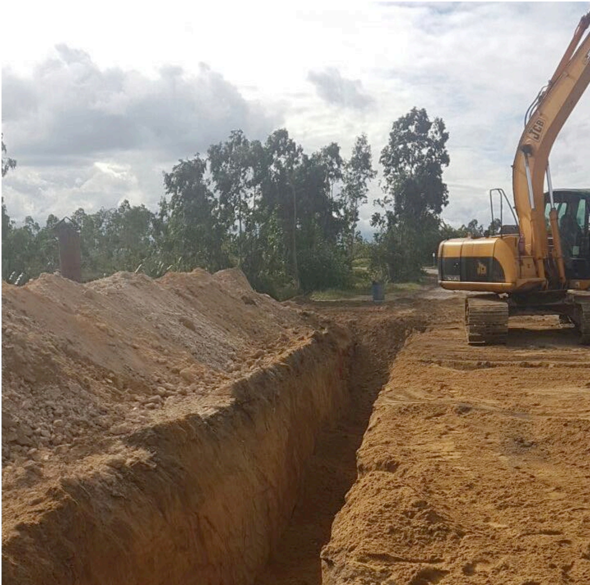
Figure 8: Trenching for installation of fibre optic Internet cable to Process Plant.
