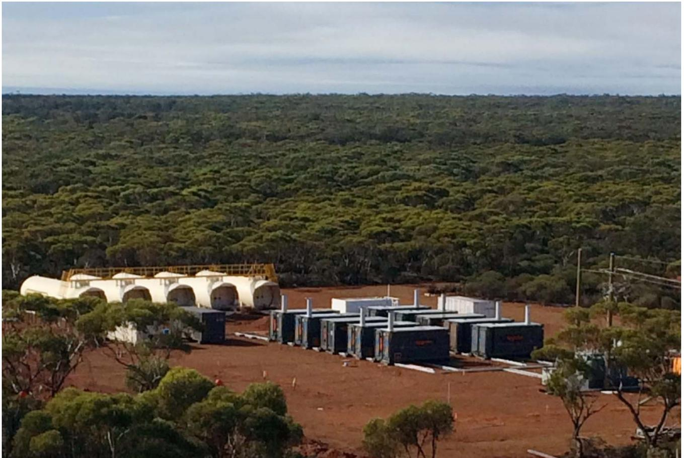
New 5.5MW containerised diesel power station and 550,000 litre fuel storage facility
