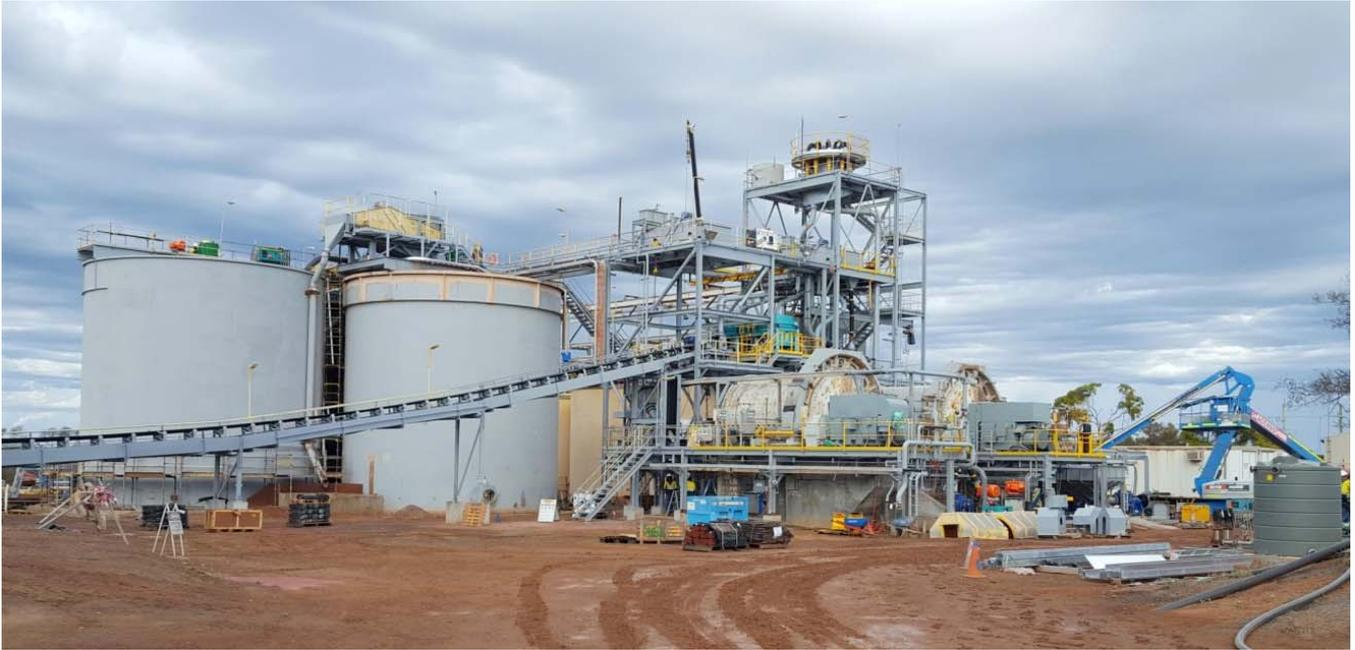
Refurbished mill feed conveyor, grinding circuit, new cyclone cluster, new gravity circuit (Nelson Concentrators coloured green) and preleach tanks.
