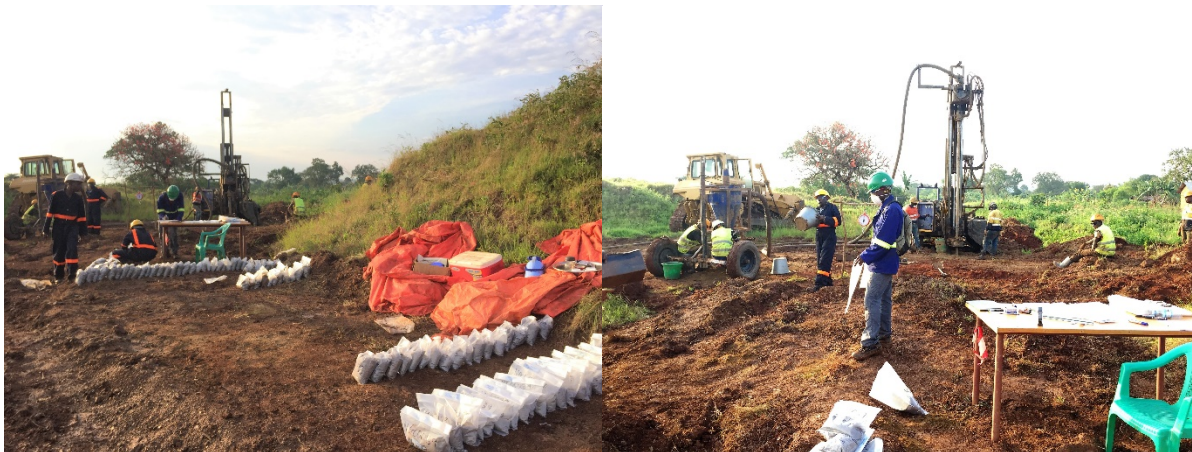
Fig 5. AC drilling and sampling in P2
