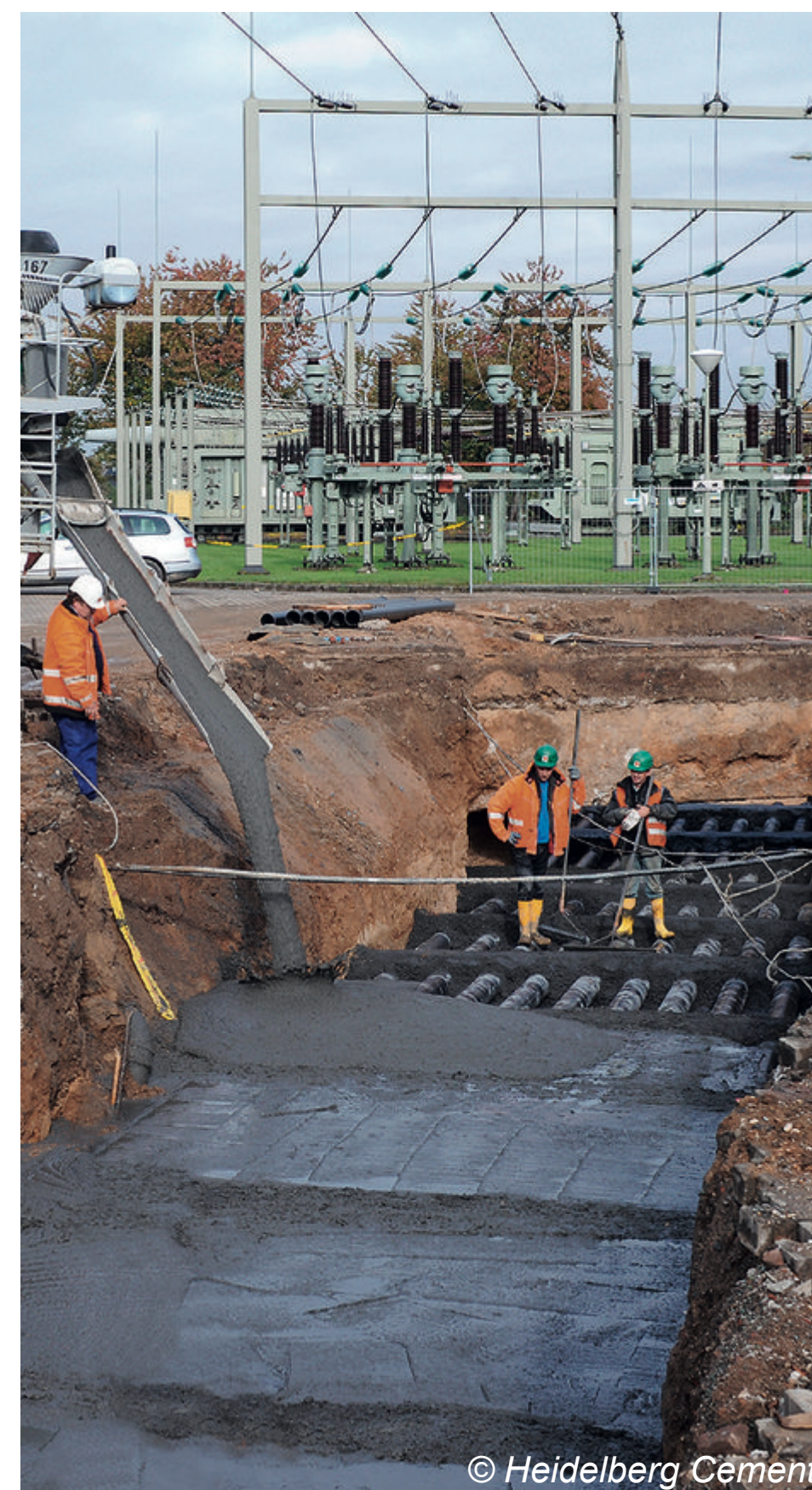
Thermal concrete in underground power line application.
