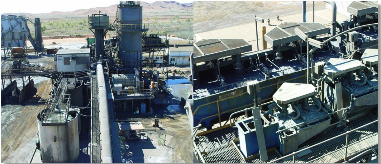
Figure 5: AGIP Radio Hill Nickel/Copper Operations (Fox 100%) – Radio Hill 425,000 tpa Treatment Plant and floatation circuits.
