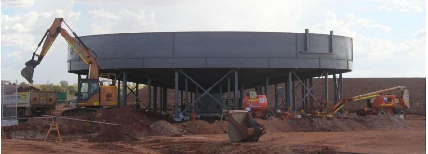
**Figure 4** – Tails thickener installation
