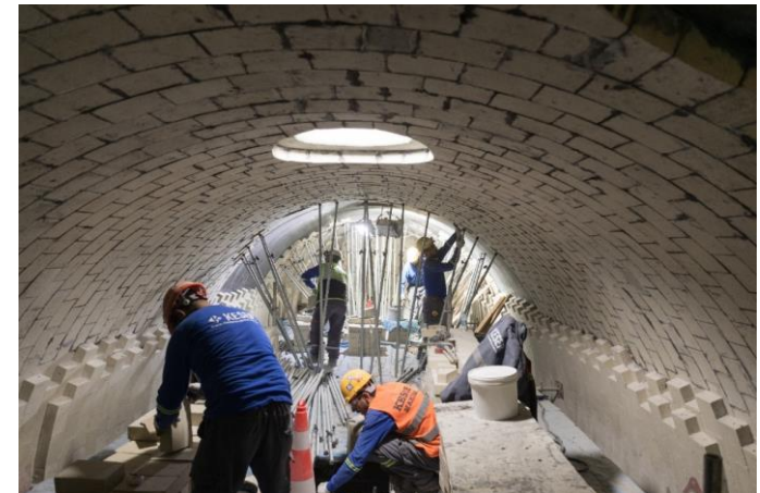
Autoclave Brick Lining
