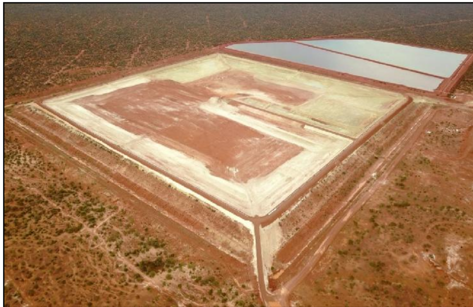
Photo 8: Dalgaranga Tailings Storage Facility (foreground) and Evaporation Ponds In Use (background)
