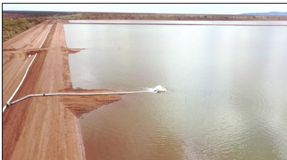
Photo 10: Evaporation Pond Cell 1 Discharge from Golden Wings, Sly Fox and Gilbeys Pits
