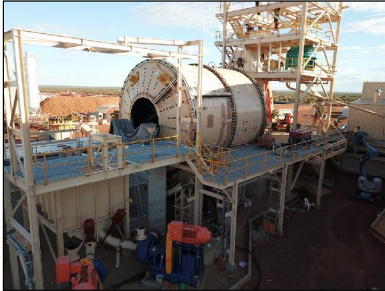
Photo 3: SAG Mill Installation – Progressing Well
