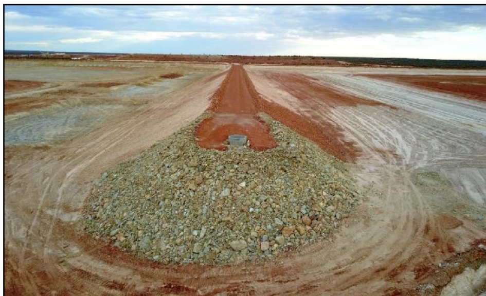
Photo 9: Dalgaranga TSF Decant Structure
