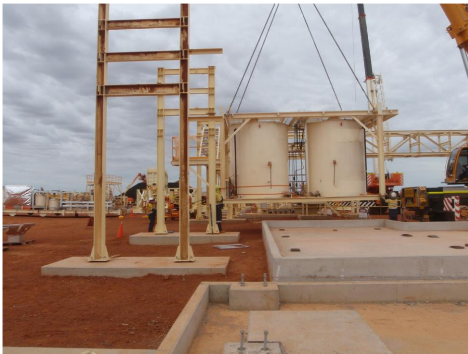
Lime make-up skid being installed
