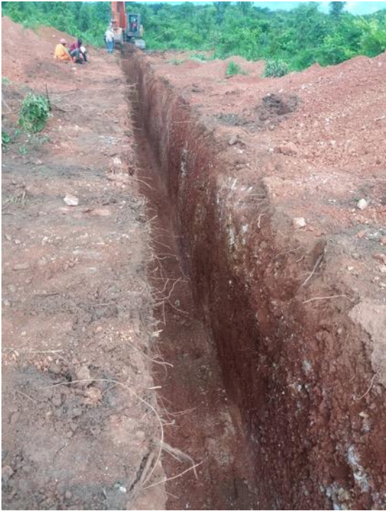
Figures 3 and 4. Trench 008 showing exposed and weathered pegmatite from surface dipping 10° to 15° west and providing upper contact structural data
