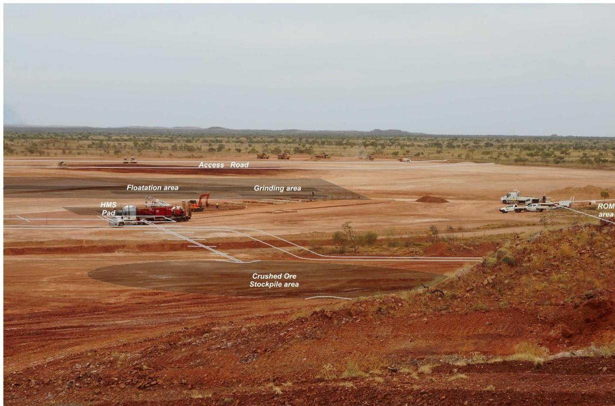
Figure 2 – Pilgangoora Process Plant Site Detail
