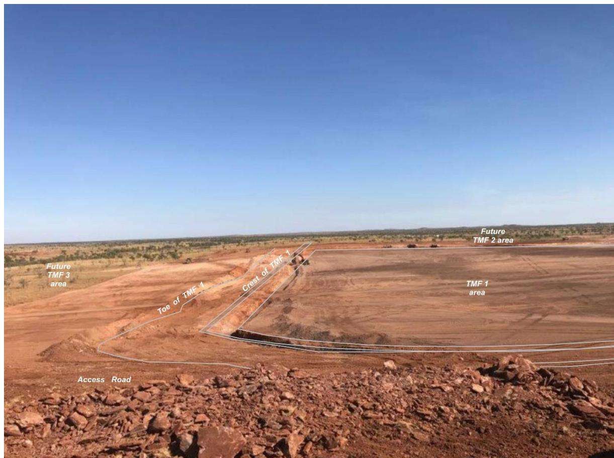
Figure 3 – Pilgangoora Tailings Dam Detail (Clearing and Cell1 Wall Key Trench)
