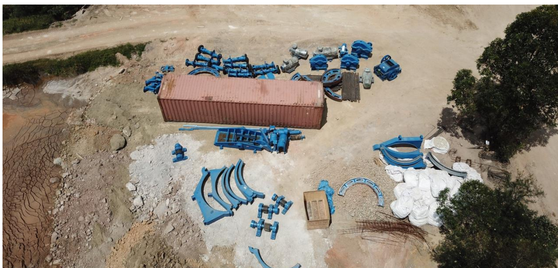
Figure 5: Major processing equipment being unloaded.
