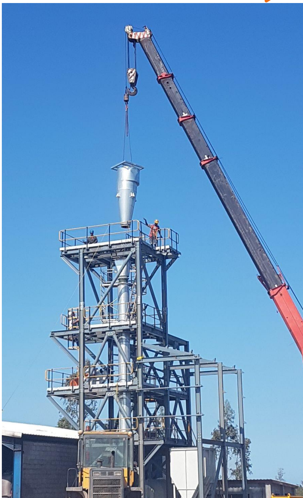
Figure 6: Cyclone installation at the MDS.
