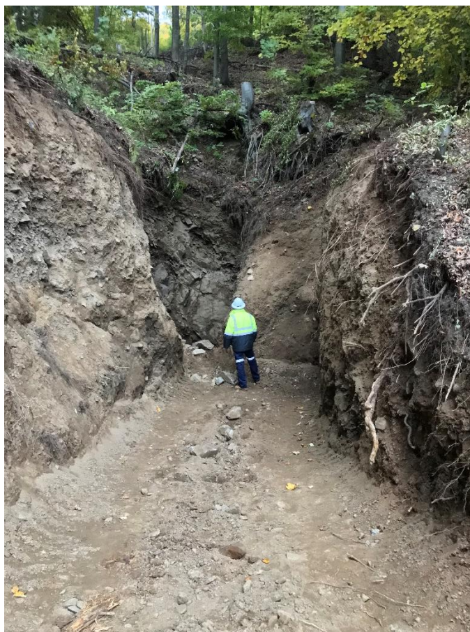
Figure 1: Joremeny Adit Entry- Box Cut Site Works
