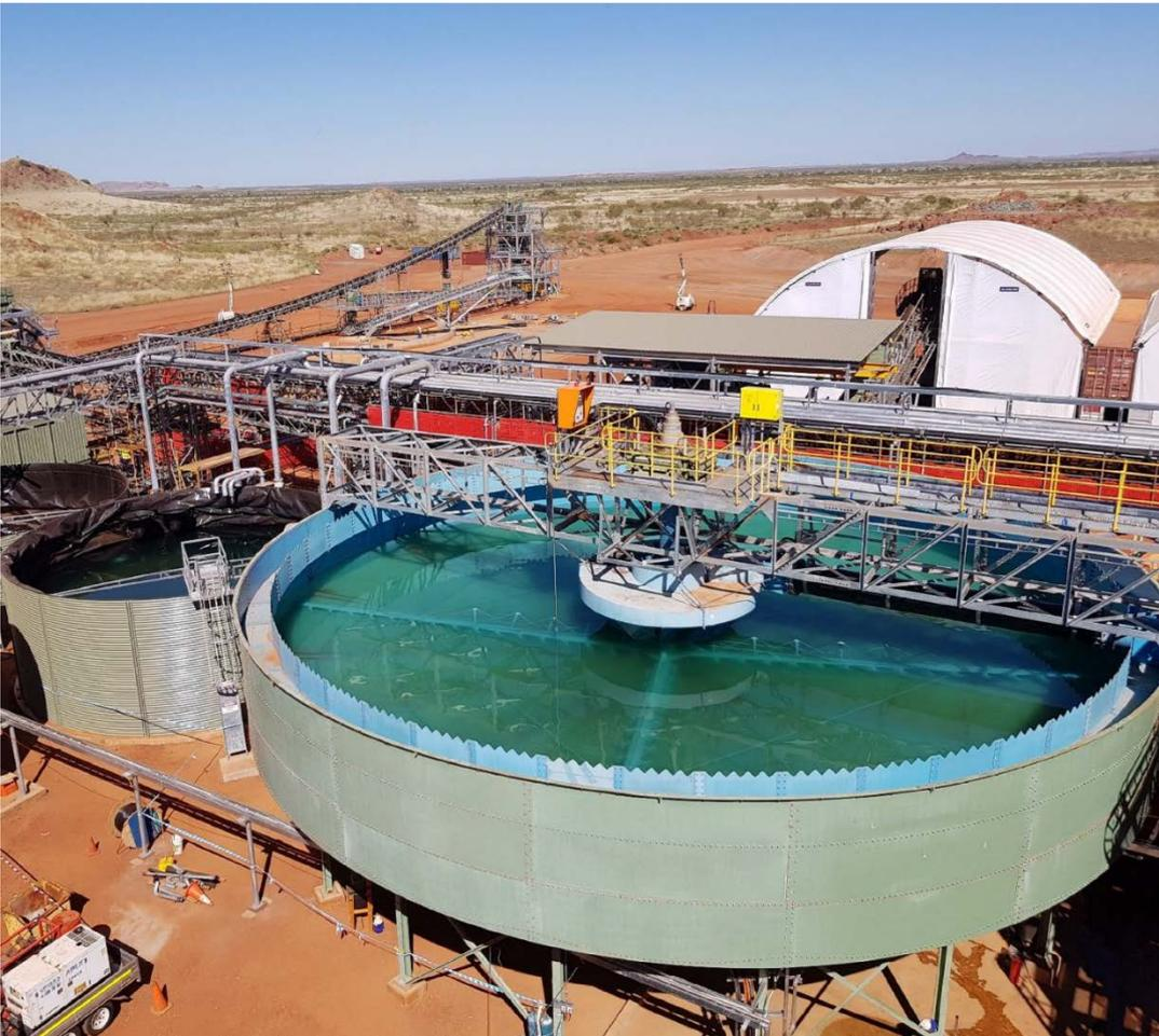
Thickener tank full of process water during wet commissioning
