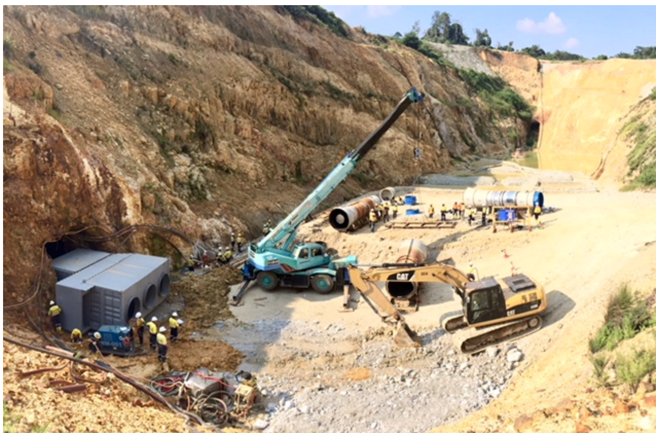
Figure 5. Installation on the new primary ventilation fan in progress
