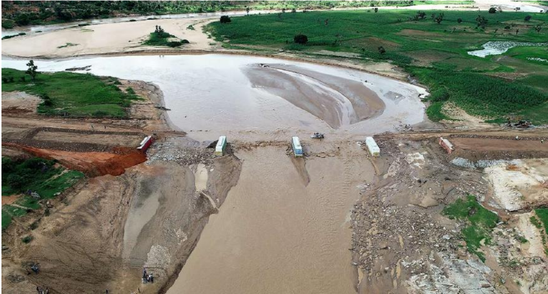
Image 2: Completed Bailey Bridge Foundations
