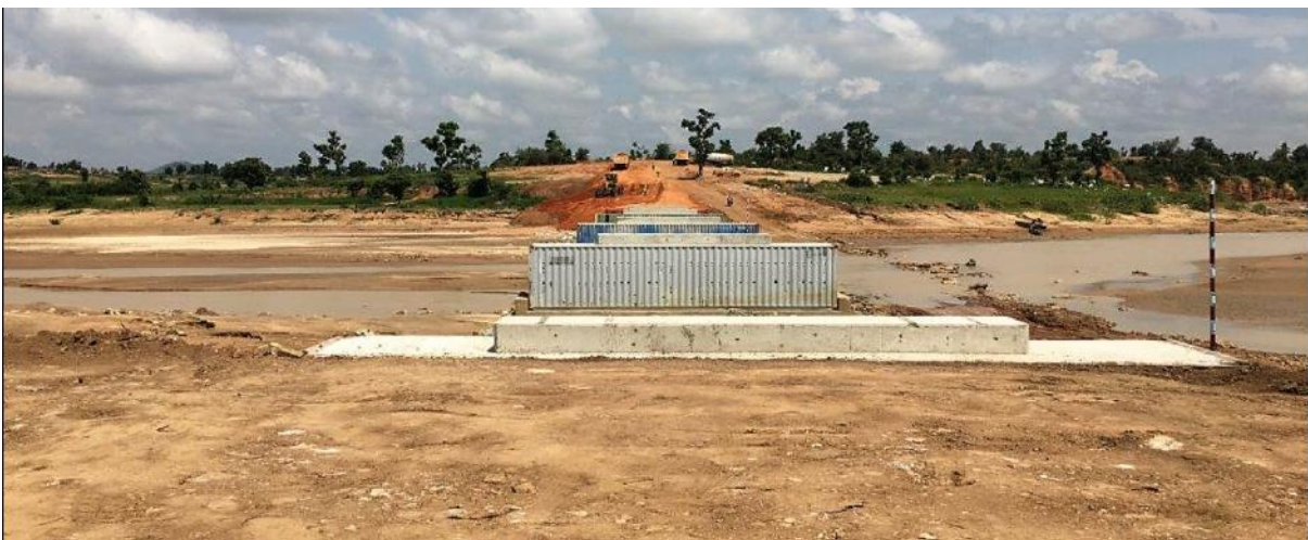
Image 3: Completion of Bailey bridge foundations
