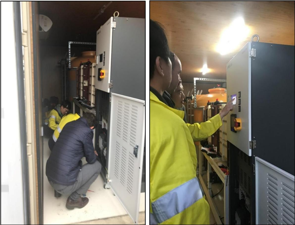
**Figure 1: KORID technicians oversee installation of the V-KOR battery at the Perth test site**
