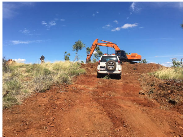
Image 6. Drill pad preparation Golden Mile.
