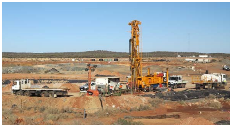
Diamond drill rig undertaking shaft footprint geotechnical drilling
