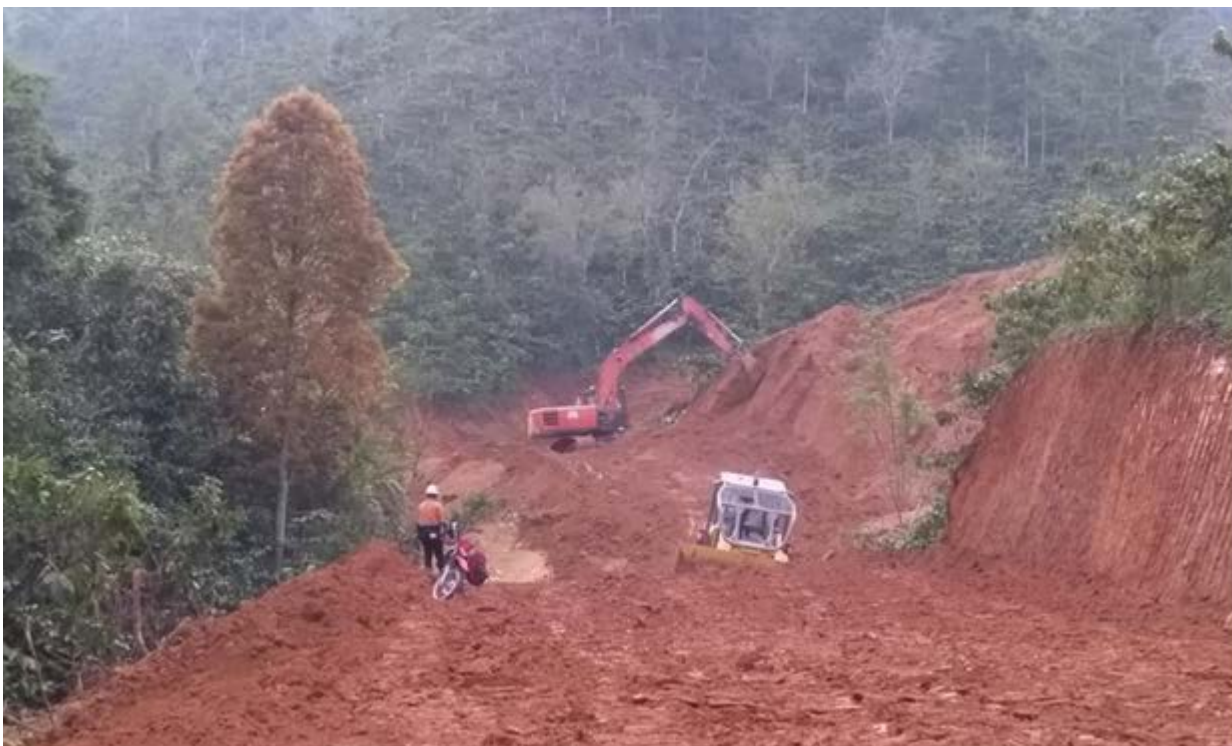
Figure 5: Topsoil Removal and Road Establishment Talang Santo
