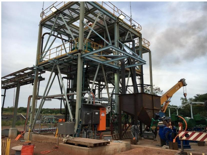
Figure 10: Syama Oxide Gravity Circuit Under Construction
