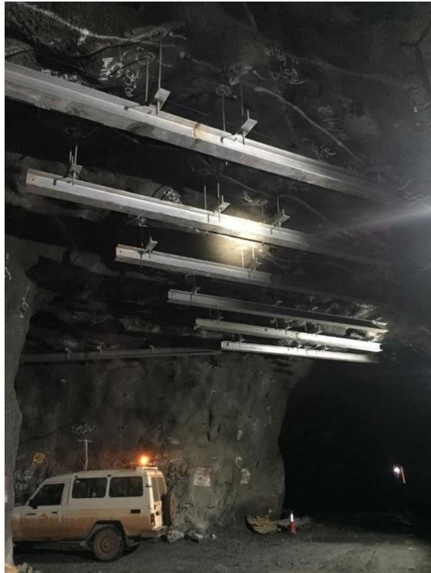
Figure 8: 1105 Pump Station Monorail Installation at Syama
