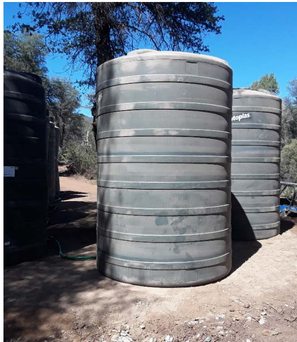
Figure 6 – Tank farm near the water well. Each tank holds up to 20,000l of water
