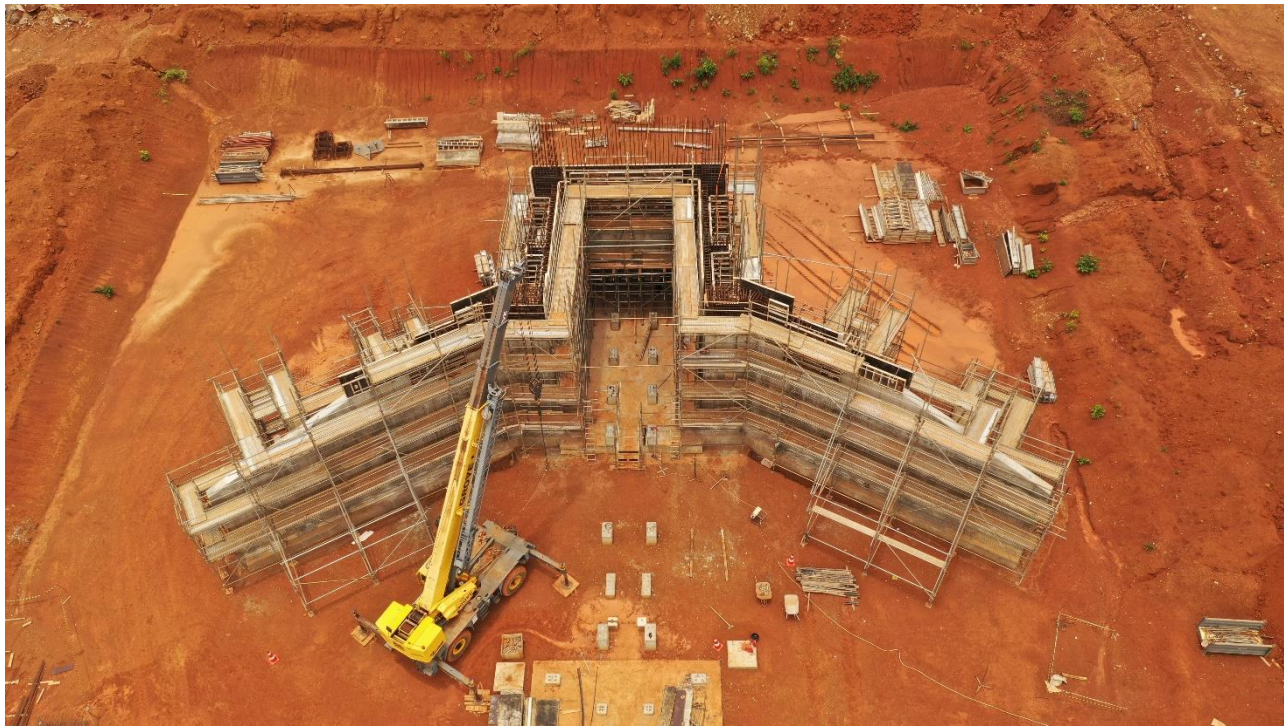
Primary Crusher Foundations
