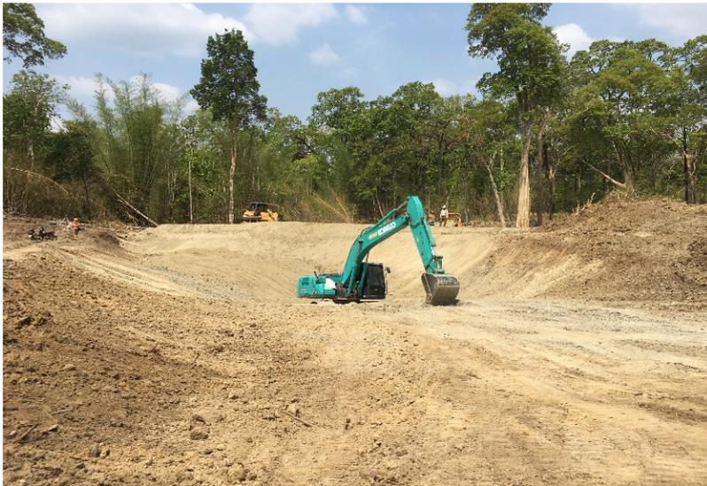
Figure 11 | Plant site cleared and topsoil pushed up following completion of geotechnical stability assessment
