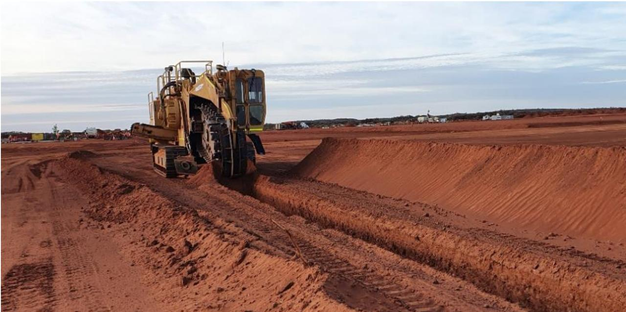
Figure 11: Excavation of trenches with a Vermeer at the Process Plant & Village site
