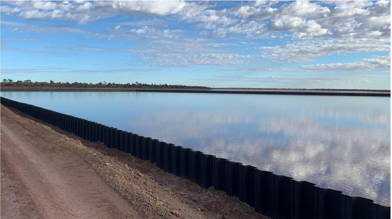
Figure 3: Stage 2 Ponds lined with PVC sheet piles
