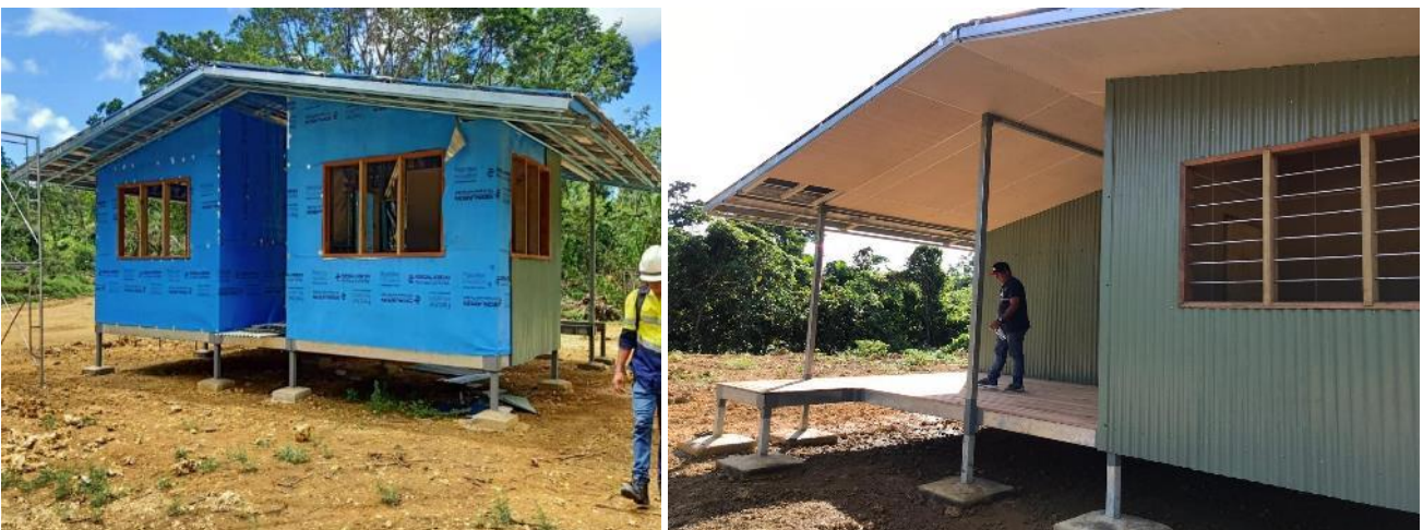
Figure 3: Construction of the new elevated steel framed houses. Modern methods are being used to replicate as much as possible the traditional style of the village houses.
