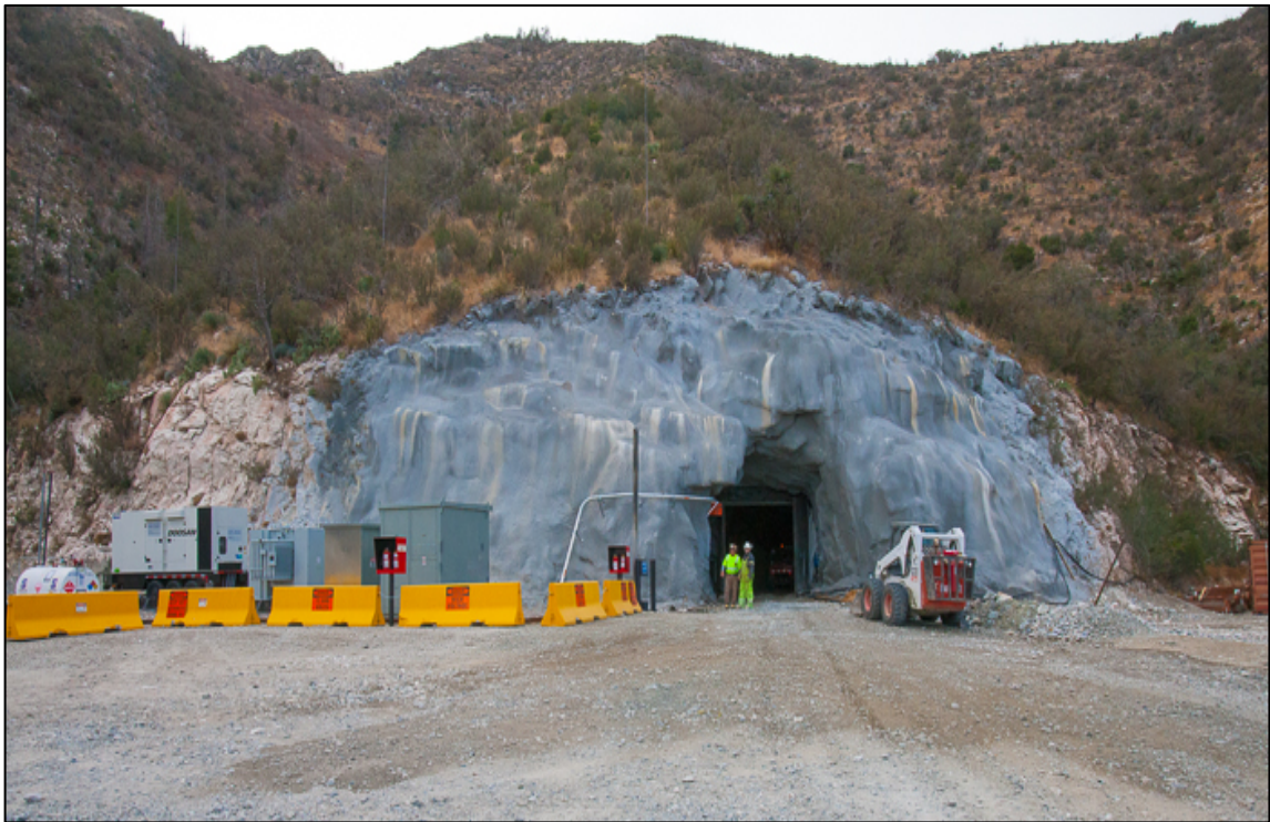
Figure 2 Refurbished 6400 Level portal with electric power infrastructure to left of portal. Note that generator shown in this photograph is currently off site
