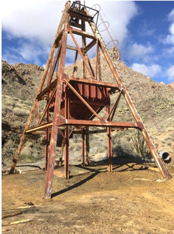
Good infrastructure is a feature of the Antler Project – the headframe, above, was used for hoisting ore during previous operations.
