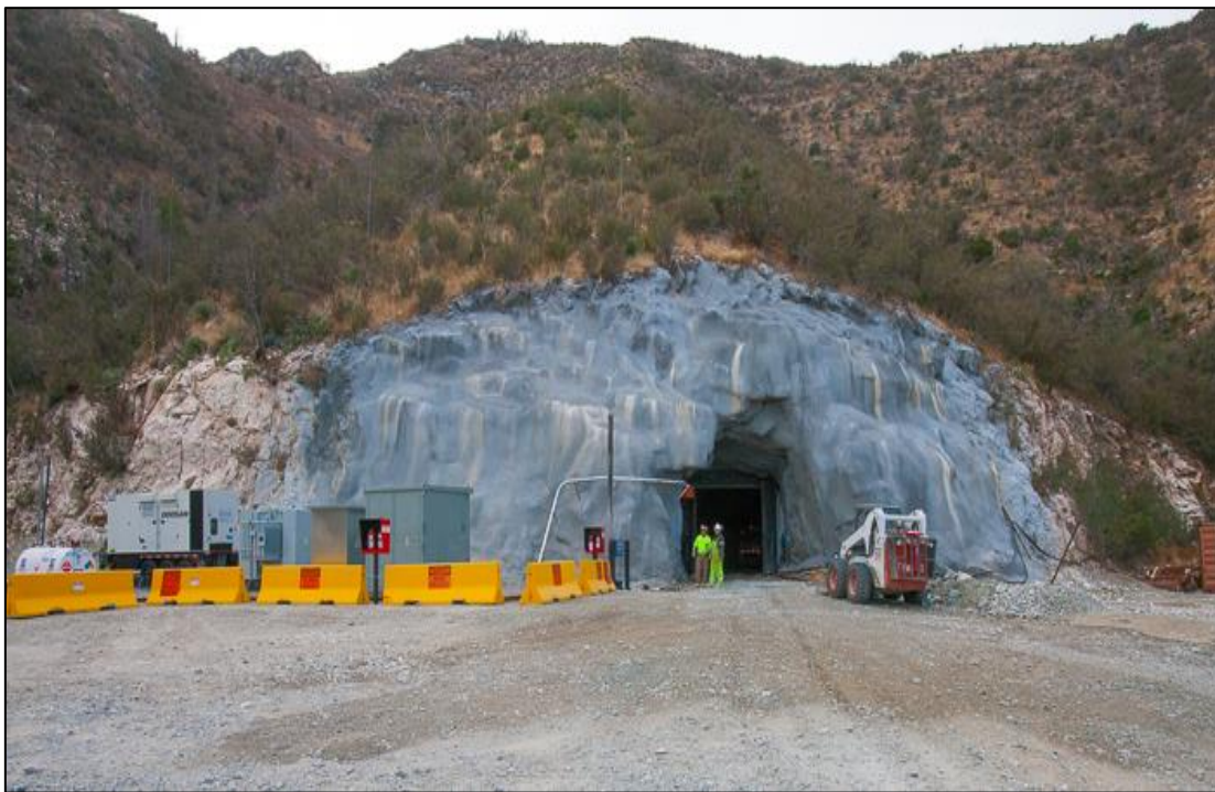
Figure 10 Refurbished 6400 Level portal with electric power infrastructure to left of portal. Note that generator shown in this photograph is currently off site
