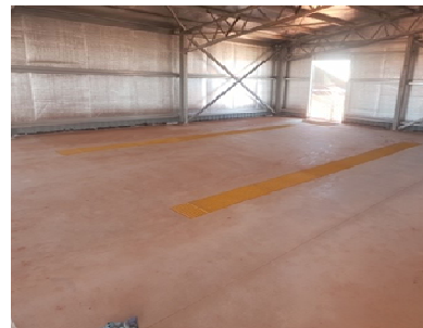
Building 1 – internal slab poured
