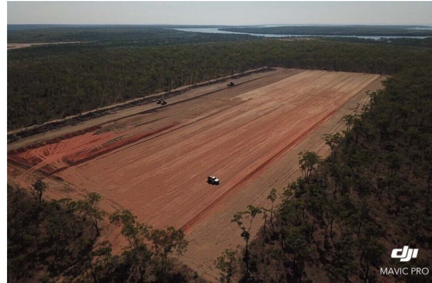
Earthworks for the processing area finished to final levels & compaction
