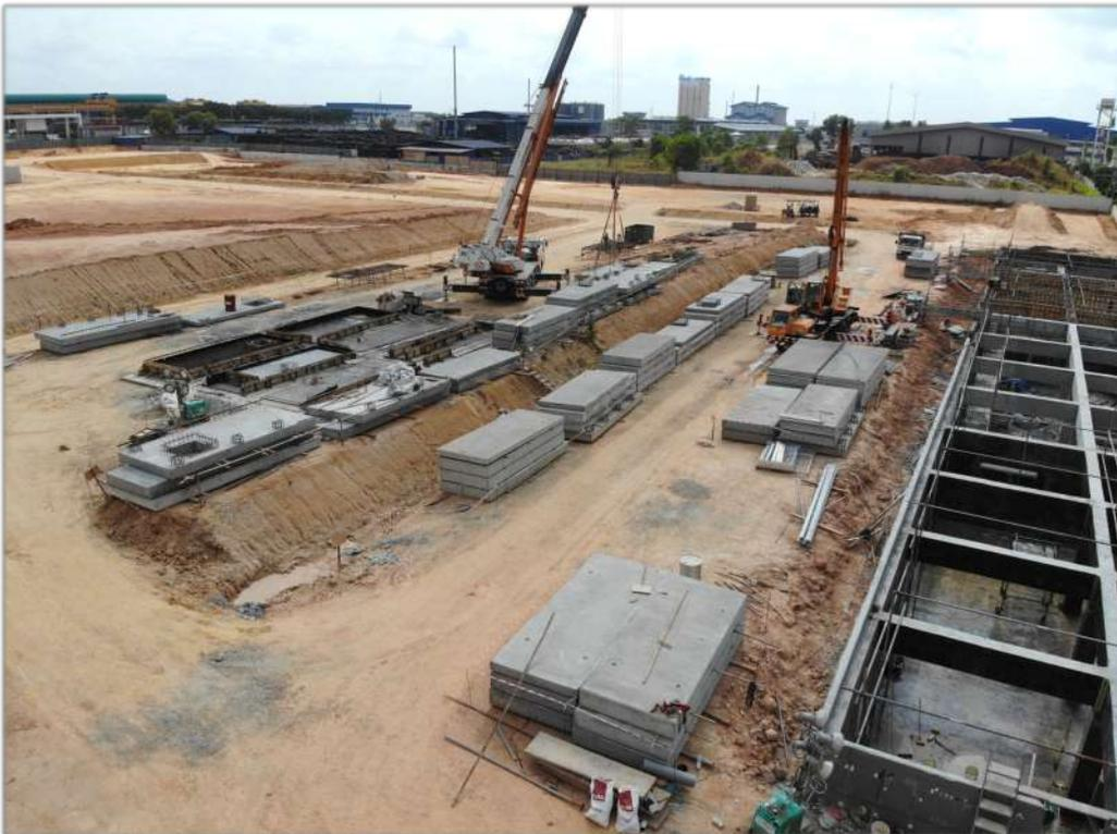
Figure 5 – OSD Tank Roof Panel Installation
