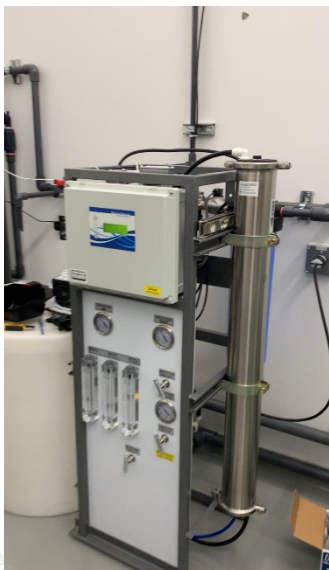
Photo 5: Global Fertigation Solutions Reverse Osmosis Water Treatment
