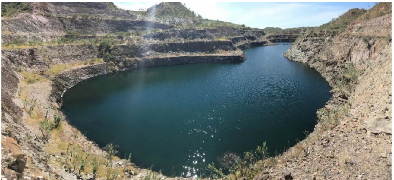
Figure 5: Butchers Creek Open Pit looking north – maximum depth 70m, average depth 30m
