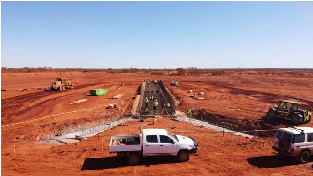
Fine ore stockpile tunnel concrete footing
