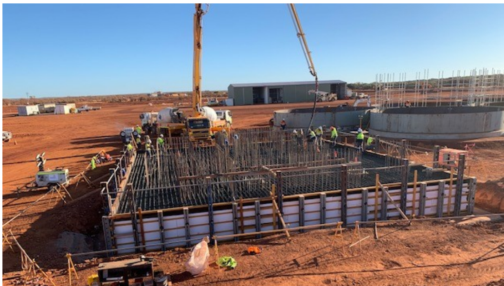
Pouring of concrete foundation for ball mill
