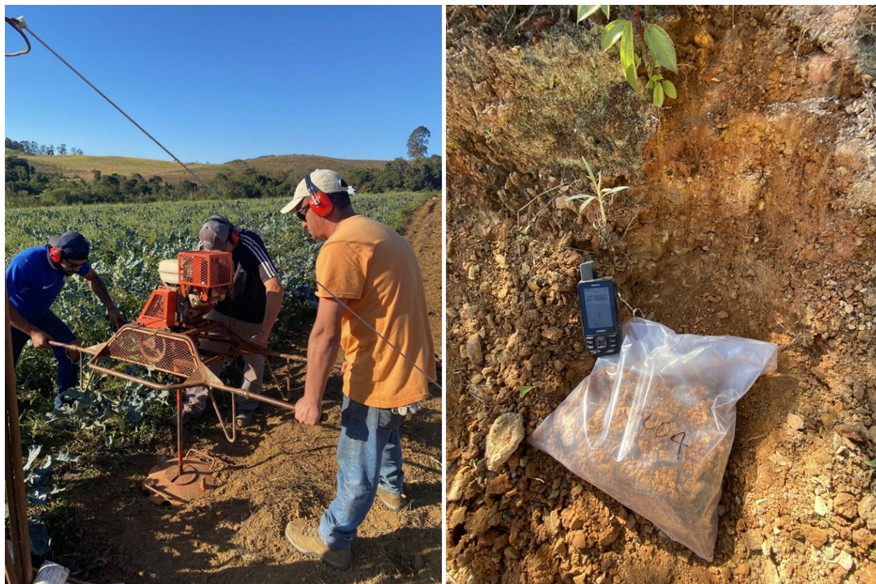
Figure 3 - Auger drilling (left) & surface sampling (right) at Raptor REE Project.
