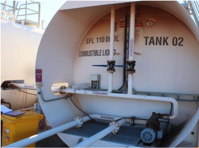
Figure 7: 110kL fuel storage tank.
