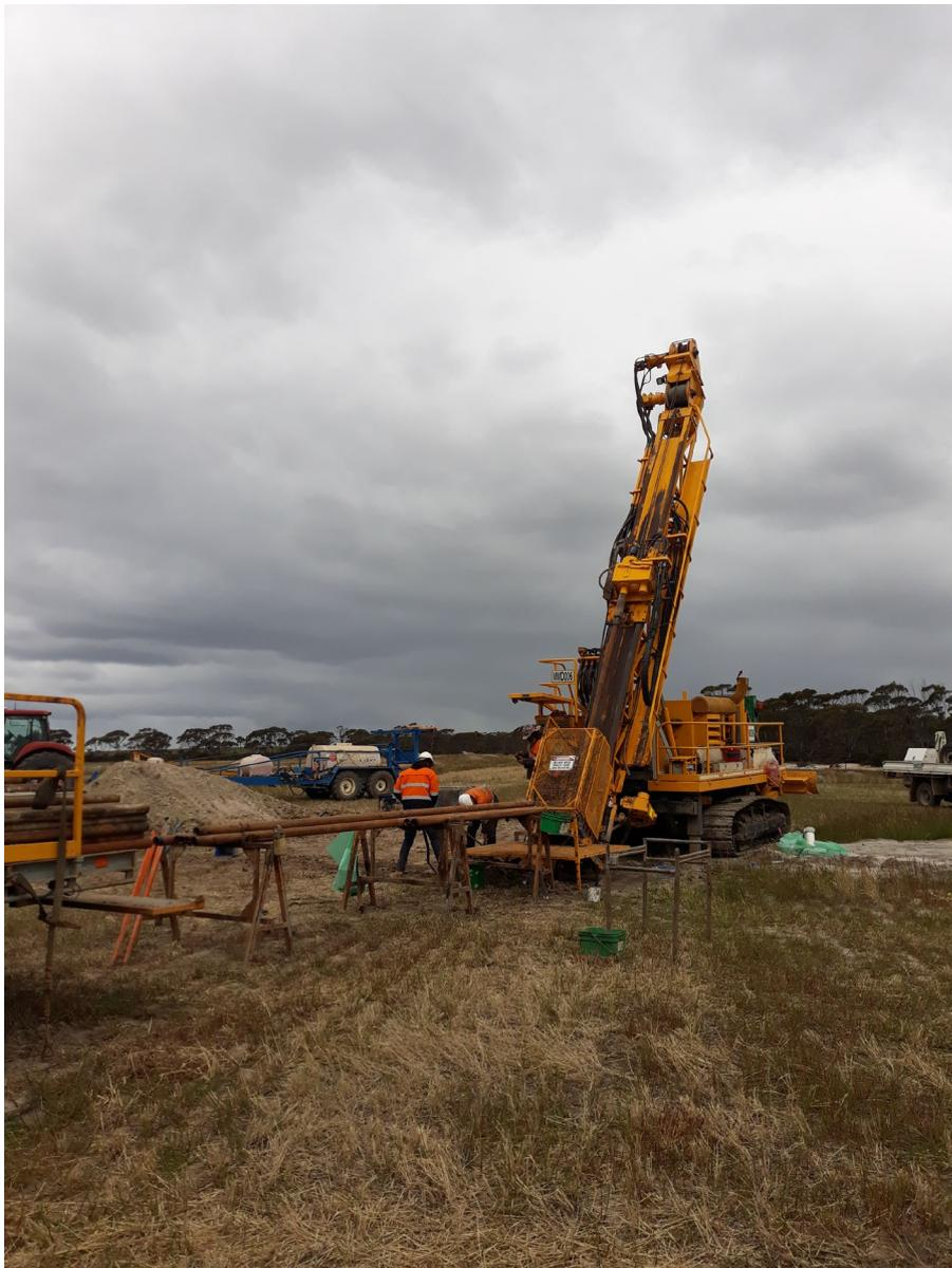
Figure 4: diamond drilling underway at Anomaly A, Circle Valley.
