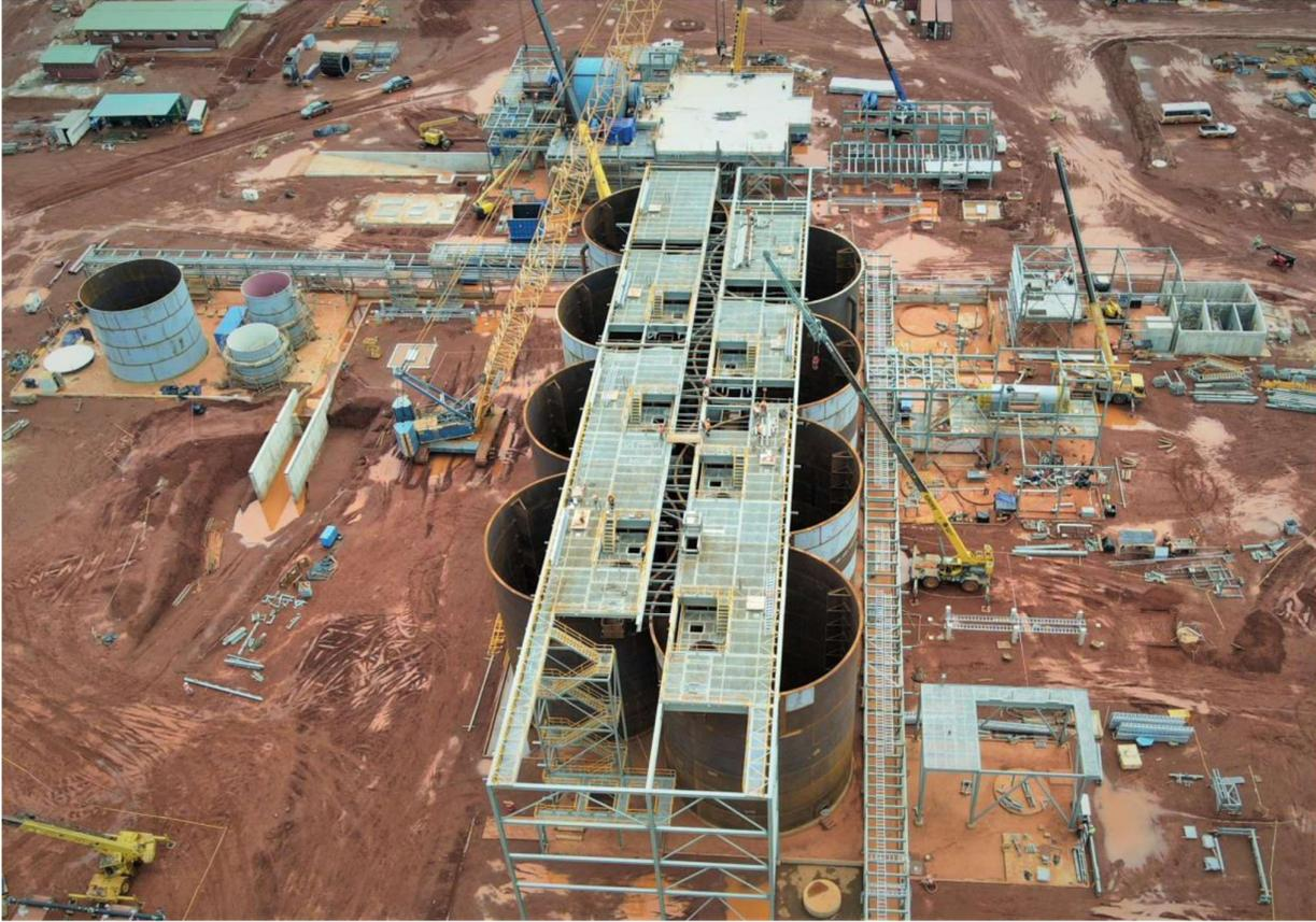
*Figure 4 CIL tanks installed*
