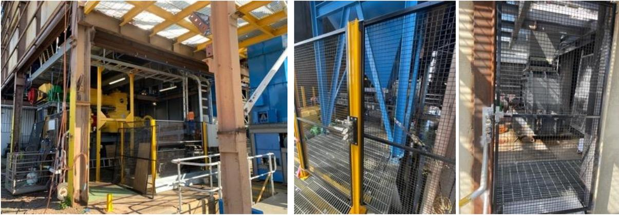
Photos (above): Installation of safety fencing.
