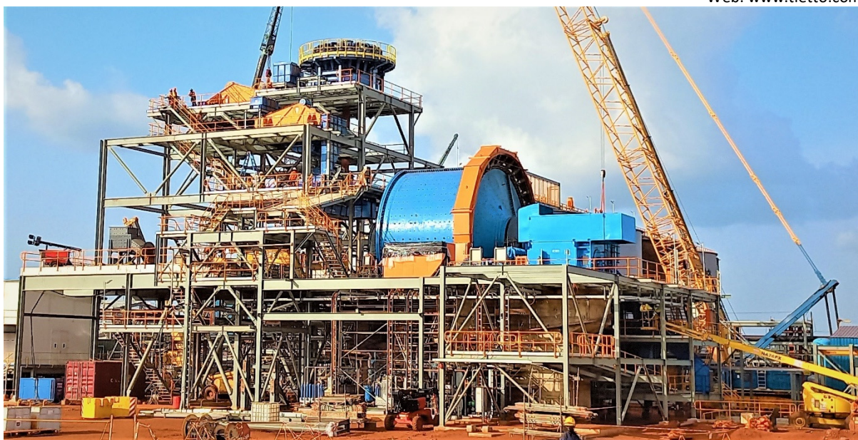
Figure 2: SAG Mill installed
