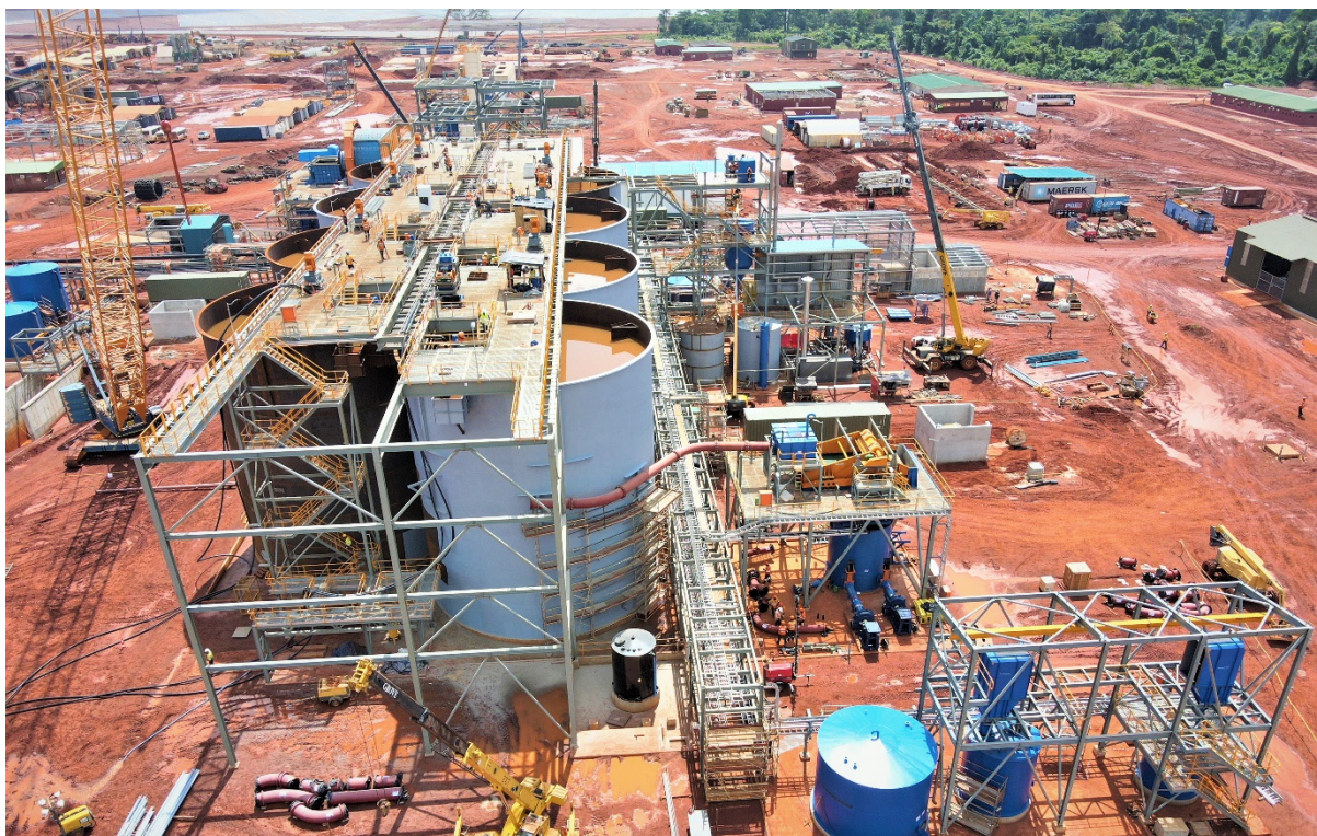
Figure 3: CIL Tanks installed and being hydrostatically tested
