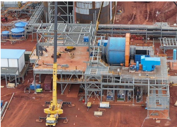
Figure 1: Overview showing construction status of the classification steel structure and CIL tanks on 7 October 2022
