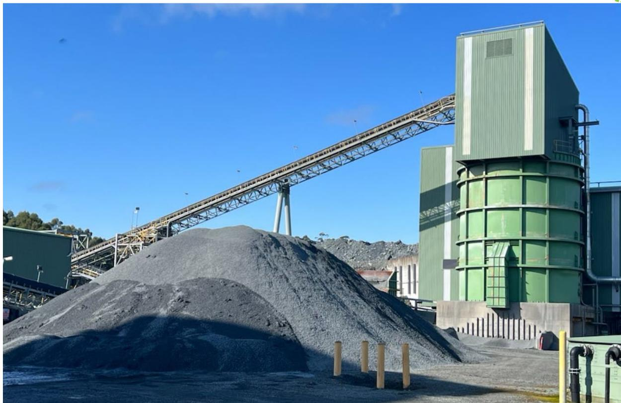
*Figure 2. Stockpile of crushed ore adjacent to the fine ore bin from the crushing circuit.*
