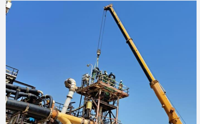
Cyclone cluster pump & pipe removal
