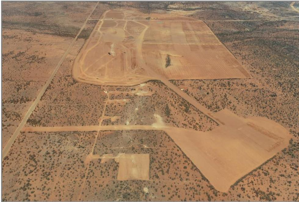
**Figure 2:** Clearing and topsoil removal well underway at Ben Hur
