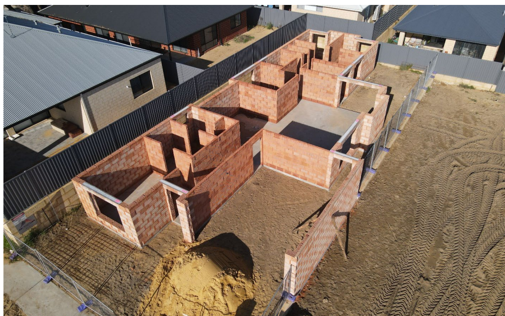
Completed structure in Wellard utilising Wienerberger Porotherm R25 & R12 clay blocks
