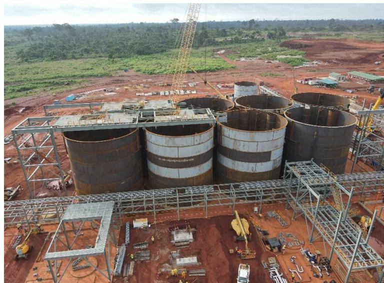
*Figure 1: Overview showing construction status of Abujar's SAG mill and CIL tanks as at 10 September 2022*
