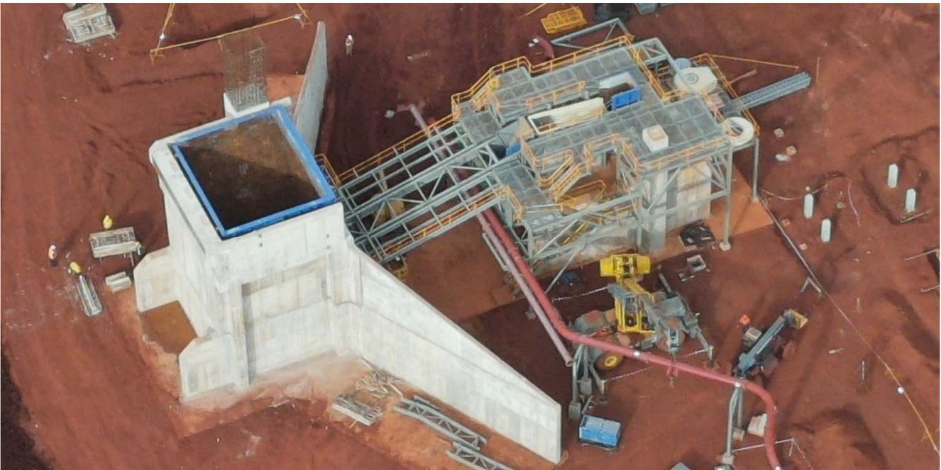
*Figure 5: Crusher installation*
